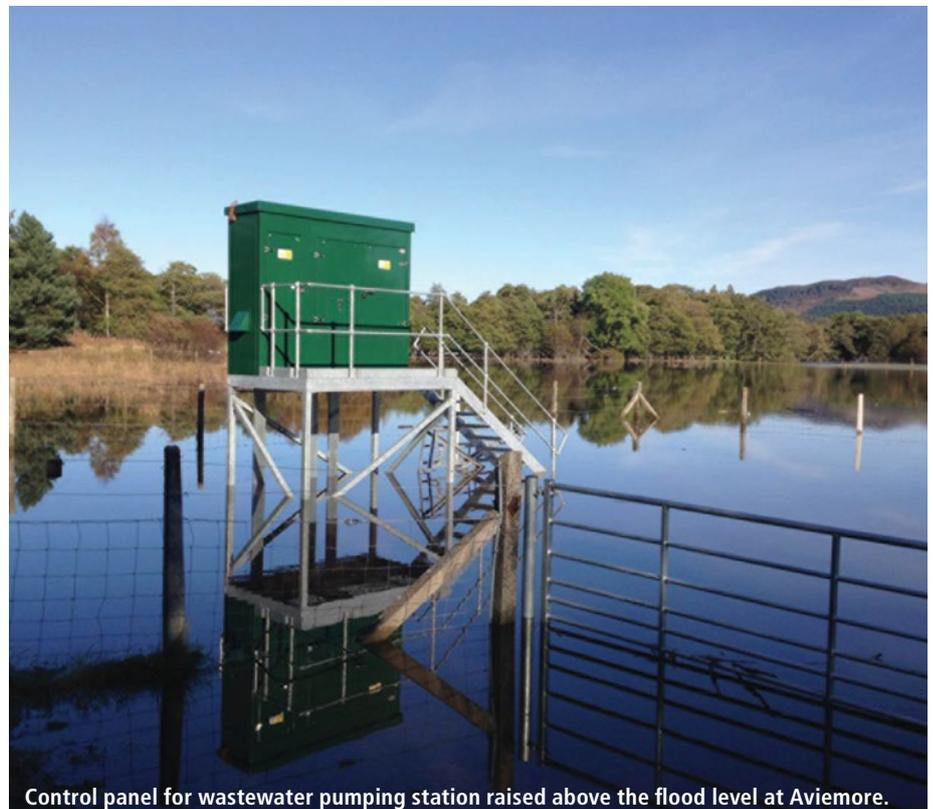
Control panel for wastewater pumping station raised above the flood level at Aviemore.
